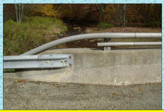
With space an issue on the guardrail, the decision is made to use the 10-inch gap at the end of the bridge.
