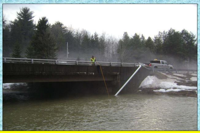
Once the arm is lowered into position, the tear drop strainer rests on the rocky stream bottom – thus supporting the pipe and taking the load off of the lowering system.
