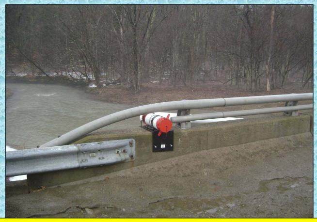
The suction head is low enough to prevent air pockets when connected to a pumper and is recessed enough to prevent snow plow damage.
