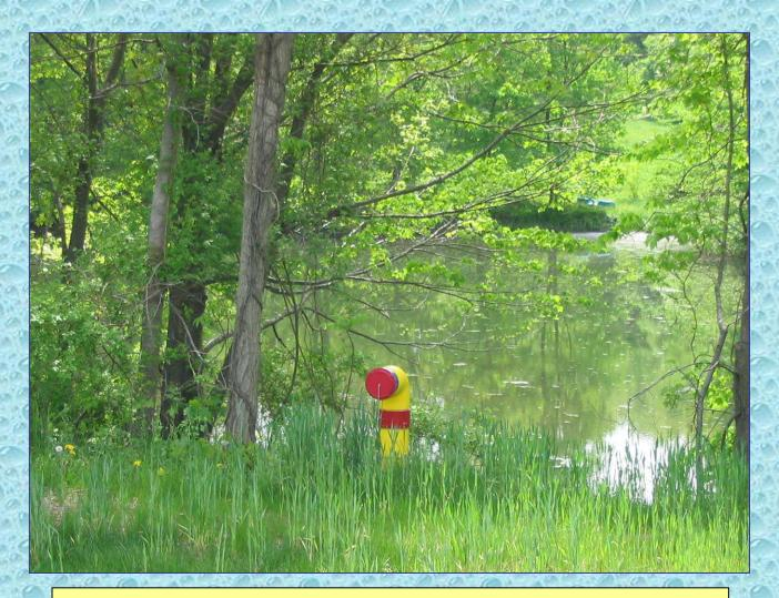
The Kochek swivel on this DFH allows more flexibility in how the engine driver positions his rig for drafting.
