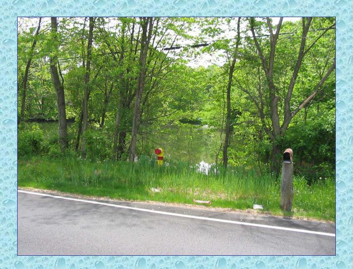
With limited access to this pond and some aquatic growth issues, the new DFH provides a means by which a pumper can get into position to take suction
