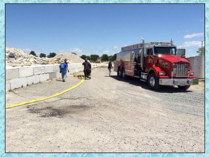
The drill started with crews executing a rural hitch operation using a 5" double-clappered siamese. Chestertown Engine 6 arrived on the scene and laid out 5-inch supply hose and went to work as the attack pumper. A few minutes behind them Tanker 6 (4000 gal) arrived and began supplying the rural hitch.
