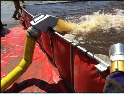
The tanker was operational by the 80-minute mark. Tankers that could not dump pumped off their water into Tanker 55 who in-turn supplied water to the dump tanks using an open relay (5-inch diffuser). Flow was moved to 1700 gpm and then again to 2000 gpm around the 108-minute mark.
