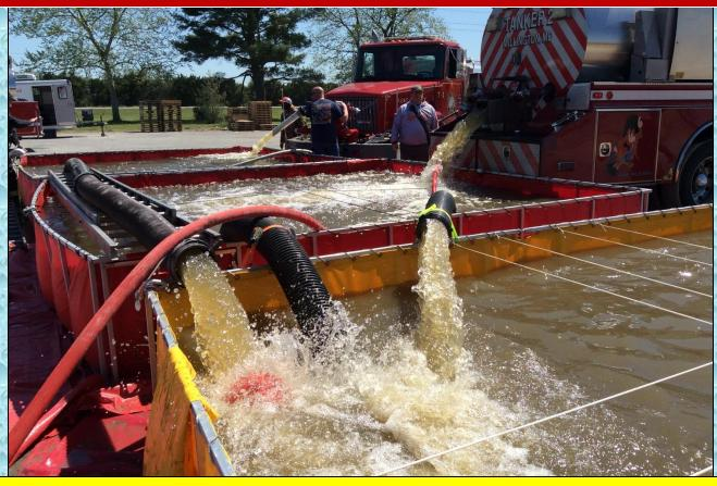
Water transfer operations became critical as flow continued to increase; this time to 1250 gpm around the 55-minute mark.
