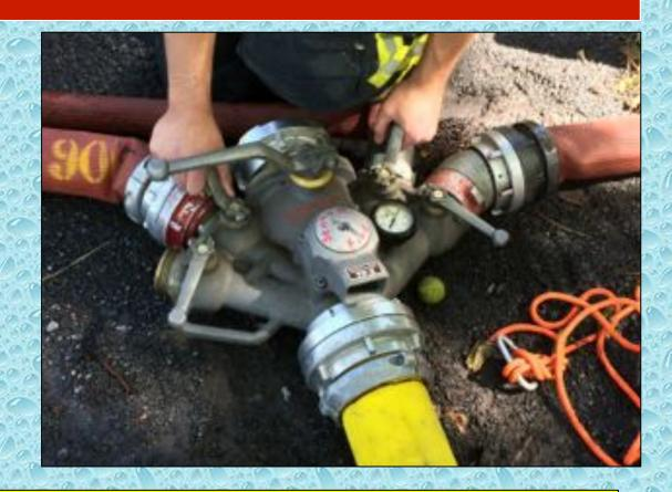
It might have been better to run a single, LDH line off of the 5" port. Better yet, turn the manifold around and use the 2.5" outlets as drains.
