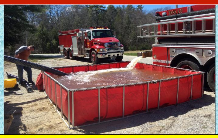
The first dump tank down was a 2500 gallon one and it was in operation by the 9-minute mark.
