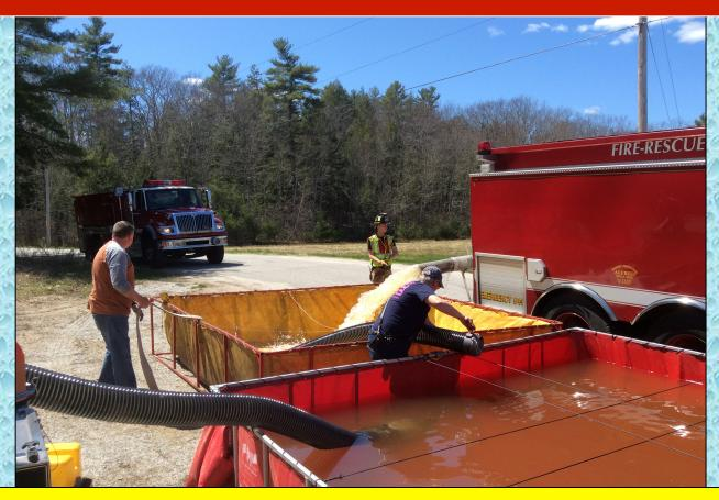
As additional units arrived on the scene, a second dump tank (2100 gal) was deployed. Water flow was started at 250 gpm at the 5-minute mark and then moved to 500 gpm at the 15-minute mark using a TFT Blitzfire device.
