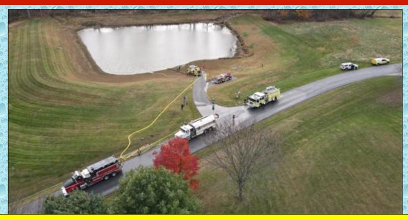
The pond was constructed for storm water management and fire protection for a local industrial park. It was renovated in 2019 and a new dry fire hydrant was installed as well as a new paved access road.
