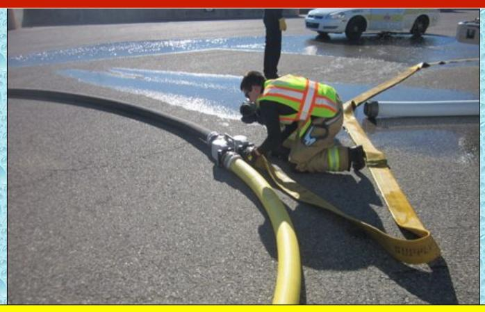
As the dump site was brought on line, the dump site engine set up to supply the other side of the double-clappered siamese – thus completing the transition.
