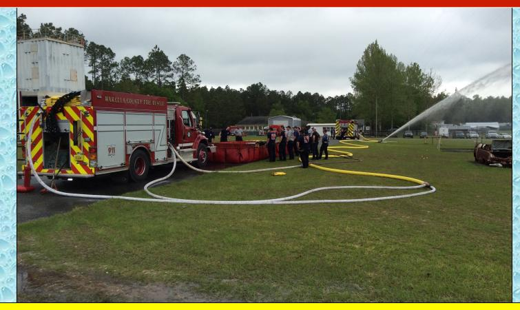
By the 60-minute mark, three dump tanks were now in use and flow was about to be increased.
