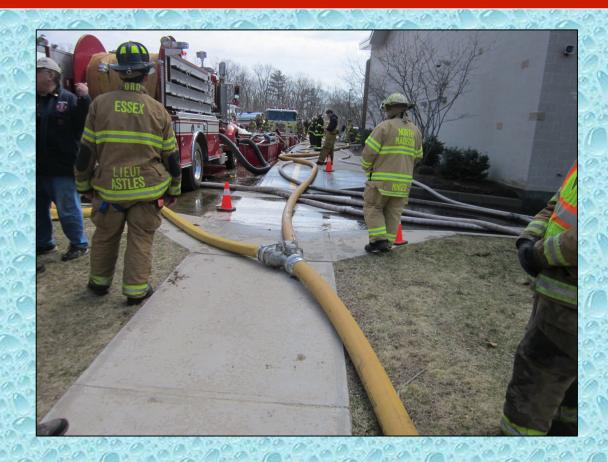
The Killingworth pumper (in the far background) supplies a 5-inch double-clappered siamese that feeds 900 feet of 5-inch to the second aerial tower.
