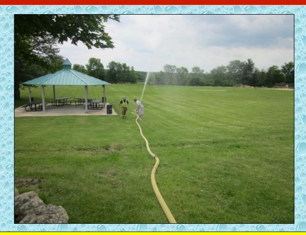
At the 5:00-minute mark, water flow was started at 250 gpm using a dump tank operation.
