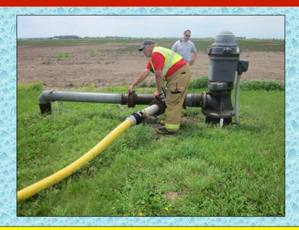
The well produced the 1,200 gpm flow at a constant pressure of 100 psi. By using 4-inch LDH – there was no need for a pumper at this fill site.
