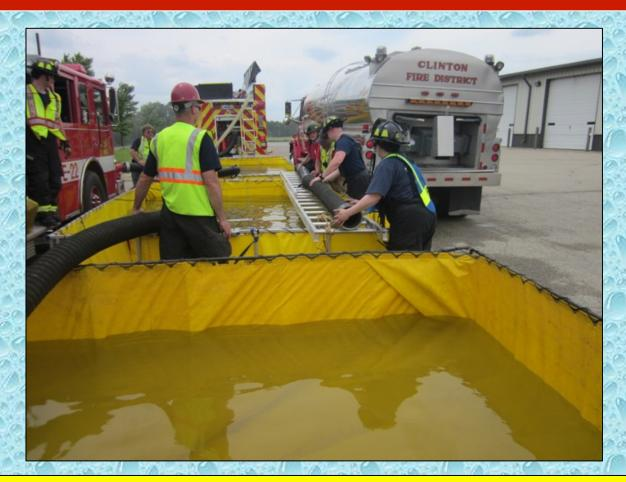
In order to transfer water quicker, crews used a ladder and additional suction hose to "jump" one of the rectangular tanks.
