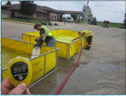
At around the 8-minute mark, water transfer operations were under way for the two dump tanks placed to the rear of Engine 51. Meanwhile, the crew worked to set up one of Fol-Da-Tank's 2,000-gallon, Single-Lane Tanks in front of Engine 51.
