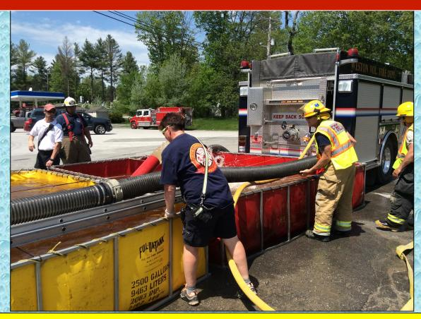
Dump site crews work to build additional jet siphons. As the flow increased at the attack pumper, the ability to transfer water at the dump site became more important.
