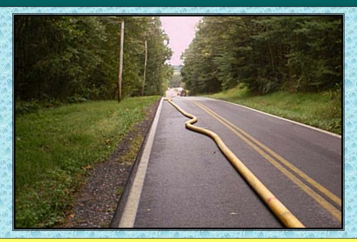
2,000 feet is a long way to move water through hose. Fortunately, 5-inch hose makes an excellent conduit – almost an above water main.
