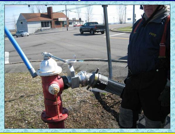
A control valve is placed on the hydrant and a hard suction hose is connected to the valve. The hydrant is turned on and the valve is turned off and only opened when needed to keep the portable tank full.
