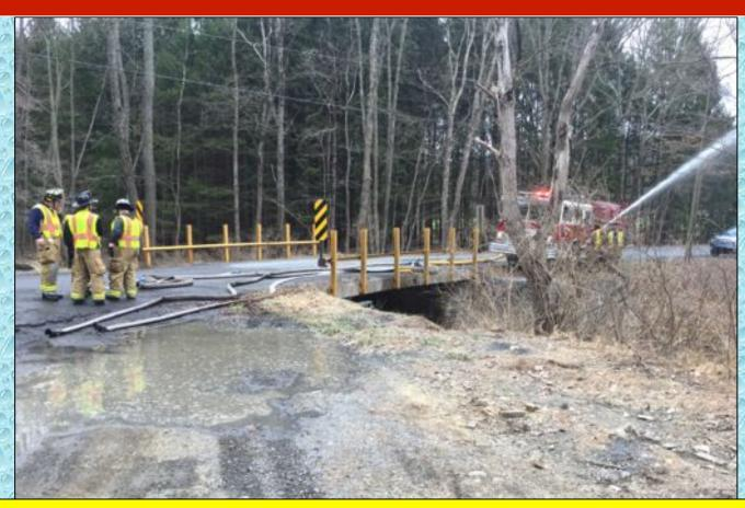
Most of the tankers were loaded using dual, 3-inch lines equipped with Storzstyle quick connect couplings. The goal was to load at 1,000 gpm.
