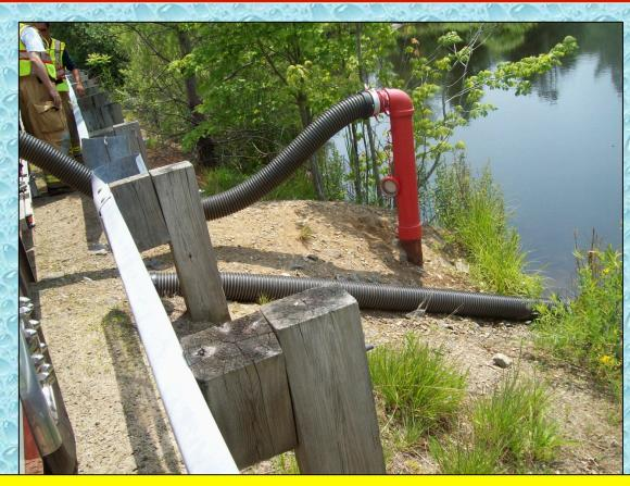
In order to maximize the capability of the 1,500 gpm pumper, two suction lines were used. The dry fire hydrant was used first and then the additional 6-inch suction line was added several minutes later.
