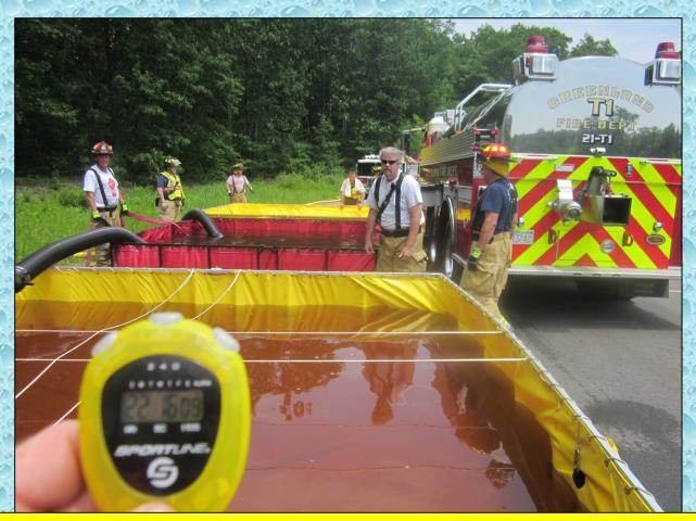
At the 22-minute mark, three dump tanks were down - with two in operation.
