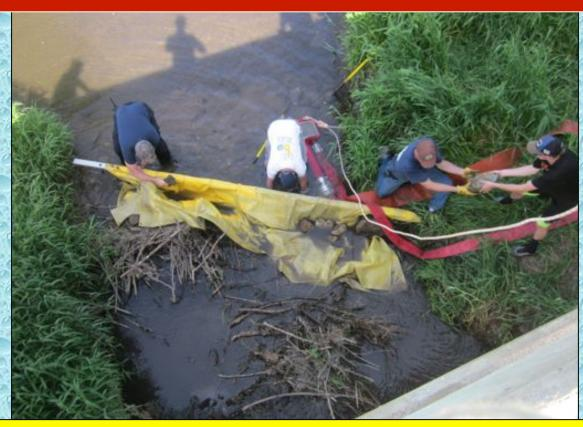
Crews had to build a dam in order to impound sufficient water for drafting. A 14-ft roof ladder and a salvage tarp were used as the base for the dam. A Turbodraft was initially used but operations were changed over to portable pumps about ¼ of the way into the drill.
