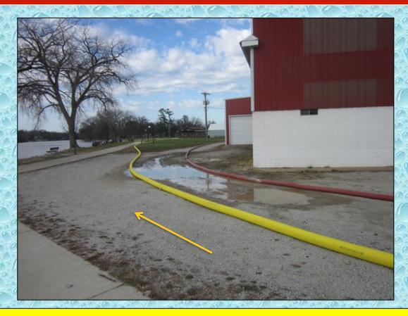
The site of the drill was a park along the river where hose could be laid out away from the supply pumper and then back to the same area – thus creating a big loop. The 6-inch (yellow) hose is going "away" from the supply source.
