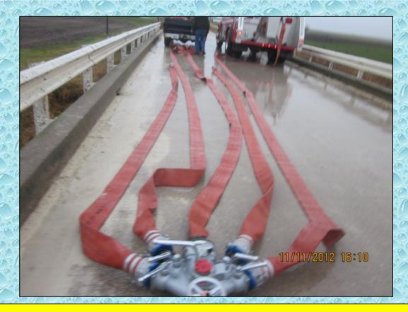
An LDH manifold was outfitted with five, 4-inch fill lines, each equipped with a cam lock style fitting.
