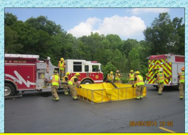
The first dump tank was down within about 2-1/2 minutes and Tanker 5 was in position to dump its water.
