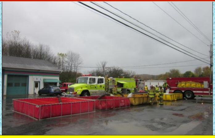
The final arrangement of dump tanks. Once the operation focused on keeping three tanks full, the 1,000 gpm flow rate was achievable.
