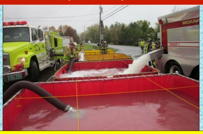
At the 84:00-minute mark, the drafting operation switched to three dump tanks with the fourth held in reserve and the flow was moved to 1,000 gpm where it stayed for the remainder of the drill.
