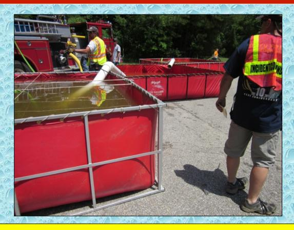
Water transfer operations are underway and the drafting problem has been resolved. Water flow to the attack pumper is back up and running at 21:23 minutes.
