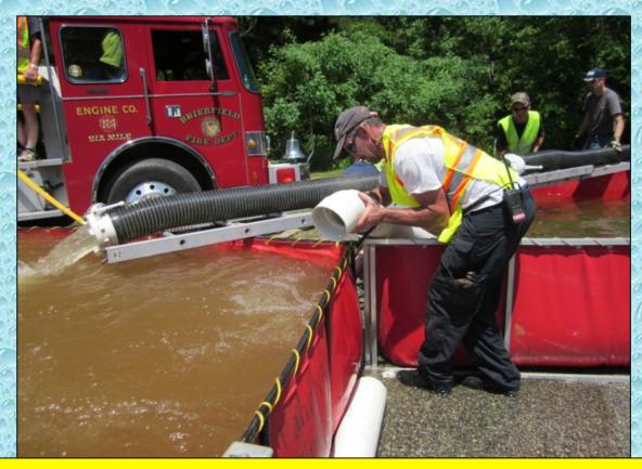
Crews worked to get additional water transfer devices up and running in hopes of getting to a 1,000 gpm flow rate.
