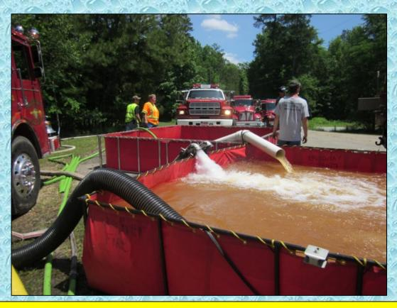
One of the issues that arose was the arrival of pumpers that could only off-load their water by pumping it off. The key was not to have them block tankers that were dumping their loads of water.
