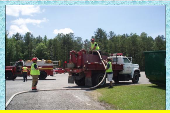
Adaptors were also an issue – a number of the tankers had different type of fill connections. The loading crew elected to just "stick" the hose in the fill tower on Vandiver's tanker – probably not the best choice because the hose staying in the tower was solely dependent on the loader being able to hold the hose in place while possibly flowing 1,000 gpm!
