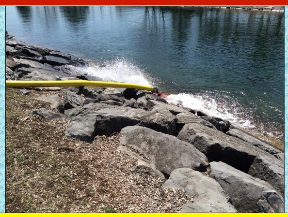
At around the 13:00 minute mark water flow was started at 900 gpm and eventually made it to 1250 gpm and then 1700 gpm near the end of the drill.
