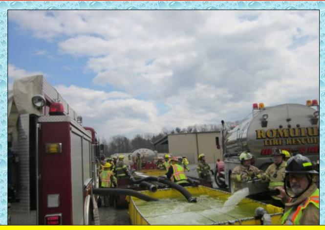
The dump site soon became a very busy place with several tankers offloading at the same time. The flow increased once again at the 58-minute mark to 924 gpm.
