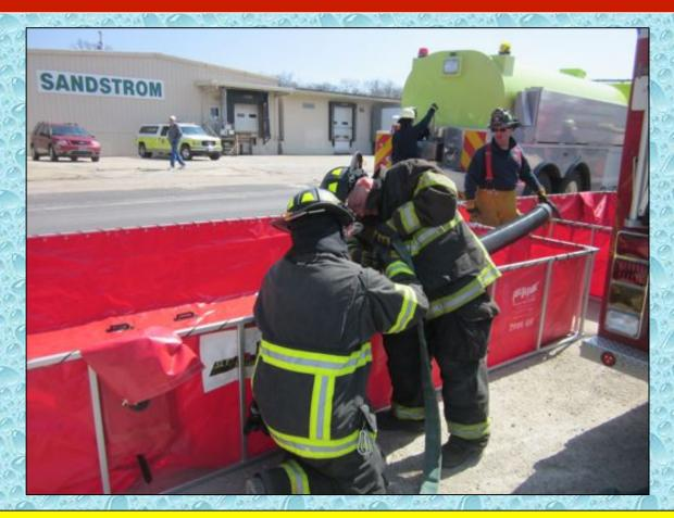
One of the critical points in the drill was the ability to transfer water to the primary dump tank. The crew is shown building a jet siphon transfer system.
