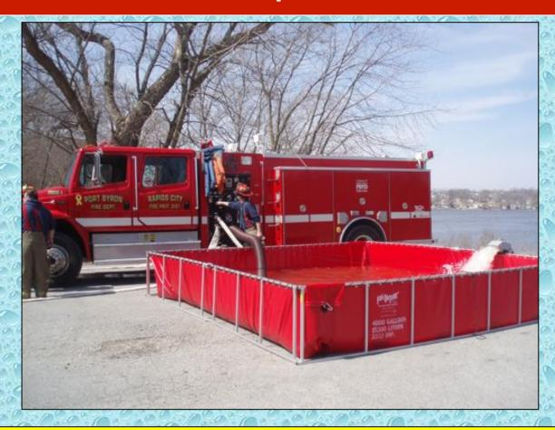
A 4,000-gallon dump tank was used as the collection reservoir for the water supplied by the floating eductor.
