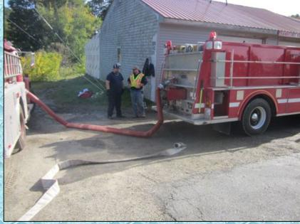
4" LDH was used to load tankers at this fill site. When possible, only the smaller (single-axle) tankers traveled to this fill site for loading.
