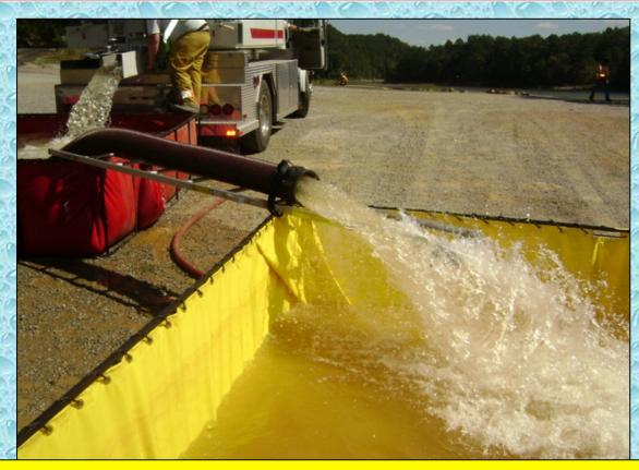
A common question asked about jet siphons is, "What pressure do you pump to the jet siphon?" The answer is simple, pump enough pressure to make the flow coming out of the jet siphon look like the one in the photo above.
