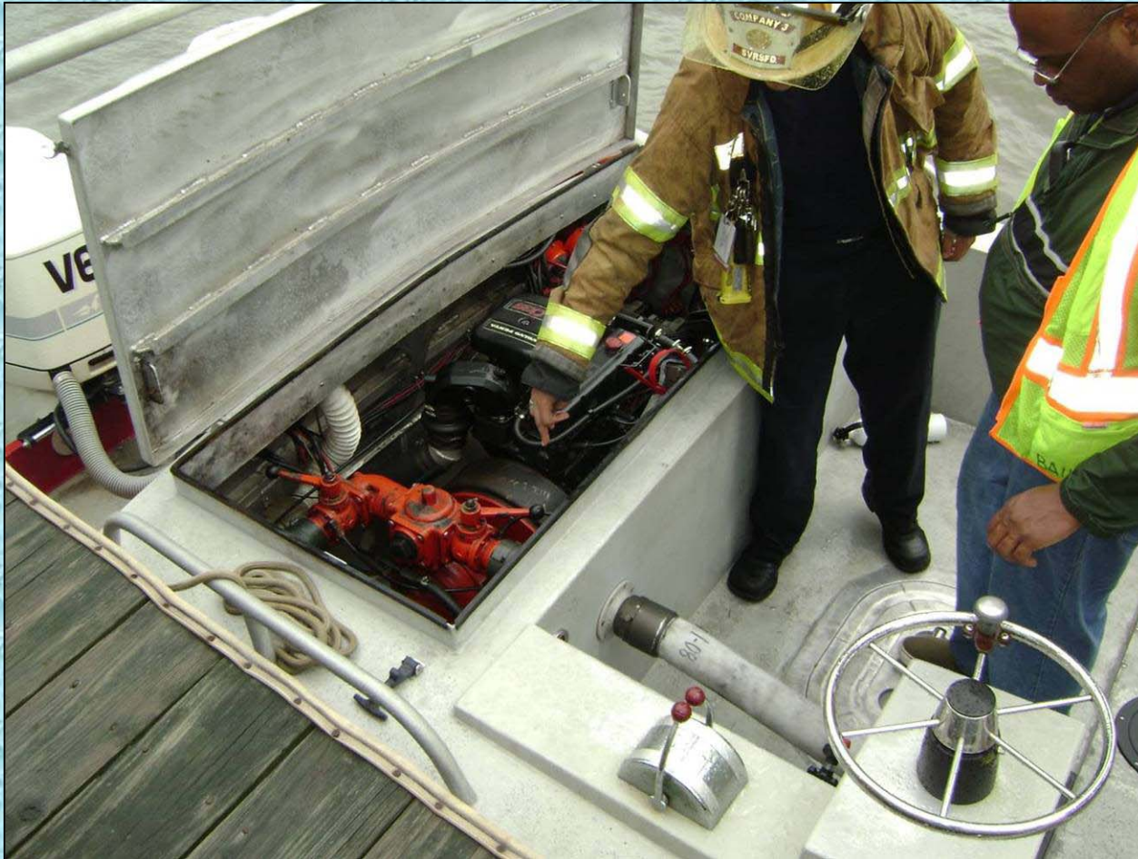
A close-up view of Fireboat 3's 750 gpm fire pump.
