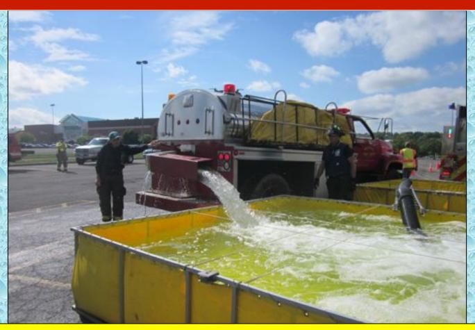
At the 38 minute mark, water flow was moved to 750 gpm and all four dump tanks were in operation.
