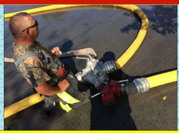
Tankers were loaded using 4-inch LDH. The crew had to get a bit creative...they built out a "valve" system that allowed water flow to be shifted once a tanker was loaded.
