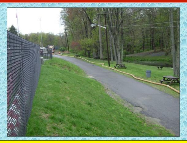
The crew laid 500-ft of 5-inch LDH from a parking lot area to the draft site so that tankers would have an easier time maneuvering in the fill area.
