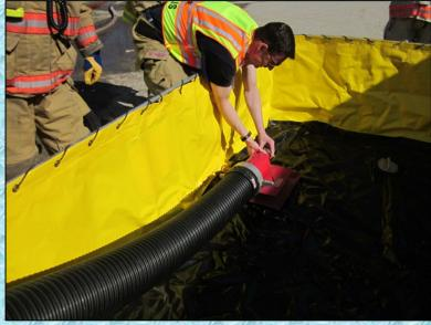
While setting up for jet siphon operations in the second dump tank, the issue of thread type arose. Seems that the 1-1-/2-inch hose had pipe thread and the jet siphon had National Standard thread – thus an adaptor was needed – which of course took some time to locate.
