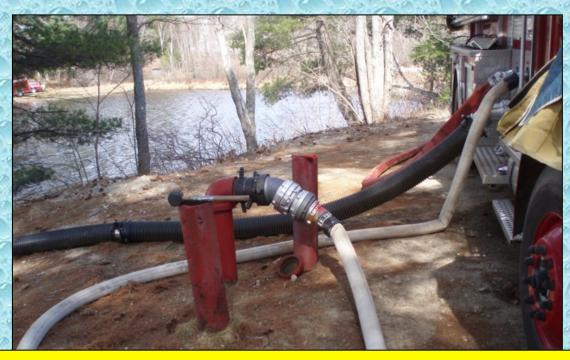
A little bit unorthodox but it worked. The Marlow crew decided to use the dry fire hydrant as their drafting circulation line. They found enough fittings and adaptors and pumped back into the dry hydrant — which actually did a nice job of flushing it out. One word of caution — this dry fire hydrant was constructed of steel pipe, and thus, pressurizing the pipe was not an issue. Crews would have to have been more careful pressurizing plastic pipe.
