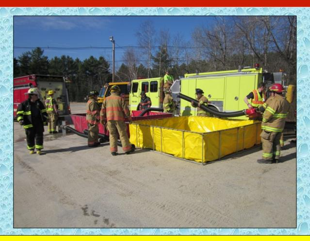
With the arrival of additional tankers, the dump site grew with the deployment of a second dump tank (1,500 gallons).
