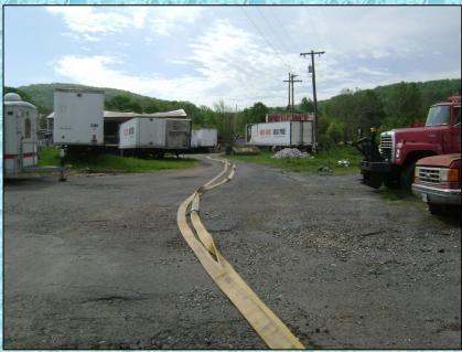
The dump site was located several hundred feet from the attack pumper and the use of 4-inch hose improved the flow capability of the operation.
