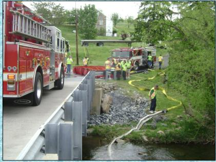
To provide additional support to dump site operations, Wolfsville's B216 (500 gpm) drafted from a nearby stream and fed Clinton's pumper.
