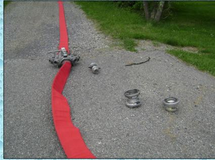
The water source for this fill site was a pond several hundred feet from the main road. The NIH rig was used to lay 5-inch LDH from the pumper at the pond to the main road where an LDH manifold was used at the loading site.
