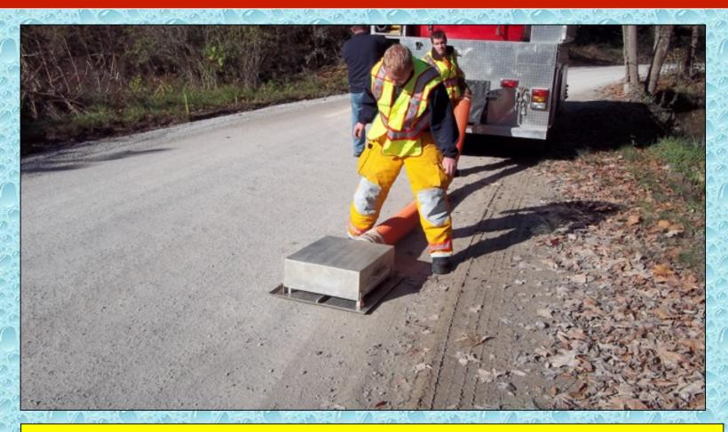
A strainer, specially designed for vacuum tanker use, is attached to the suction hose.
