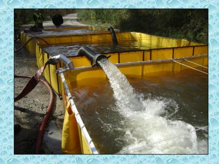
Because the portable pump cannot develop enough pressure to run a jet siphon, it is set up to float in the fourth tank and pump water to the primary drafting tank using a short length of hose.
