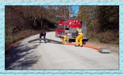
The participants for the drill were from seven different fire departments in the Boone and Lincoln Counties area and the water hauling apparatus was representative of the type of water supply support that would respond to a structure fire in the Morrisvale area.
