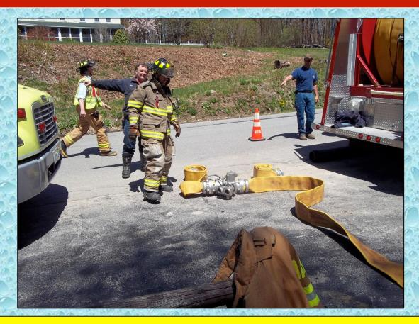
The tanker loading station was set up using 4-inch LDH and an LDH manifold. The use of LDH almost always improves tanker loading times.
