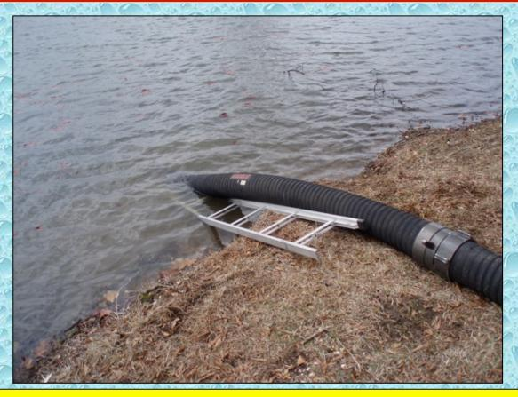
A folding ladder was used to keep the barrel strainer off the bottom of the lake so that flow would not be obstructed.
