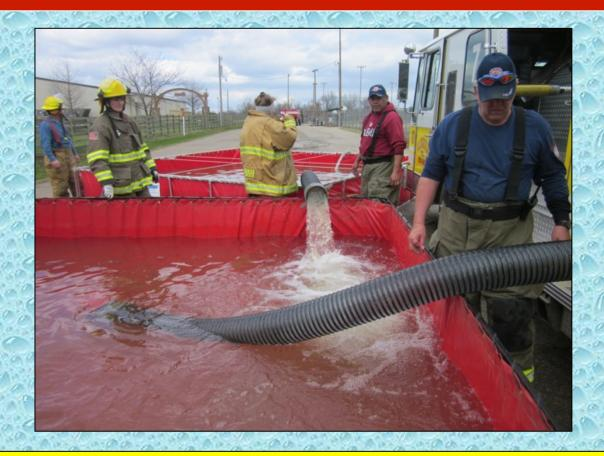
At the 11:25-minute mark, two dump tanks are now in operation. Note the "good looking" water transfer operation in place.
