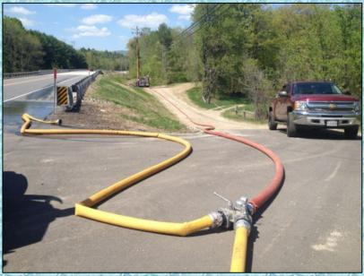
Orford Engine 3 (1,250 gpm) was used to draft from the river via a dry fire hydrant and supply 4-inch LDH to load tankers. A jumbo wye was used as the control valve for loading the tankers.
