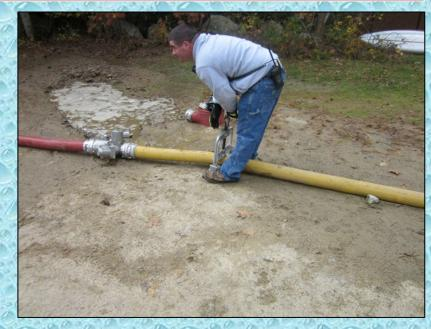
A problem occurred at the manifold being supplied by the East Andover pumper. The valve would not close all the way, so corrective action was needed to fix the problem. An LDH hose clamp was used as the flow control device – not ideal – but it worked given the resources that were available.
