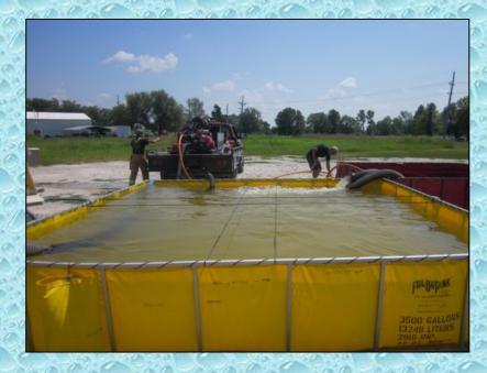
Water transfer operations were handled by the dump site pumper and by the Cutler grass rig. A total of three jet siphons were used to transfer water.
