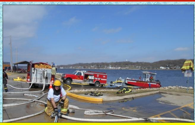
The fire boat and the pumper both took suction from the same boat ramp area. The pumper (Le Claire E5) had attempted to use a dry hydrant at the launch area but the pumper could not obtain a draft through the DFH – so the crew changed location.
