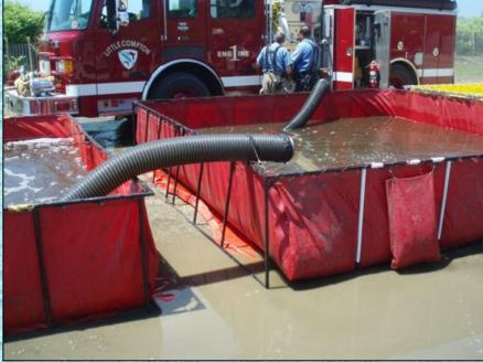
This drill featured two different kinds of siphons. The tube on the left is a Holley tube which seemed to move a lot of water and could get down very low in the tank. However, it could not "throw" the water laterally as easily as the traditional jet siphon pictured on the right. The crews knew this and spaced the tanks accordingly.
