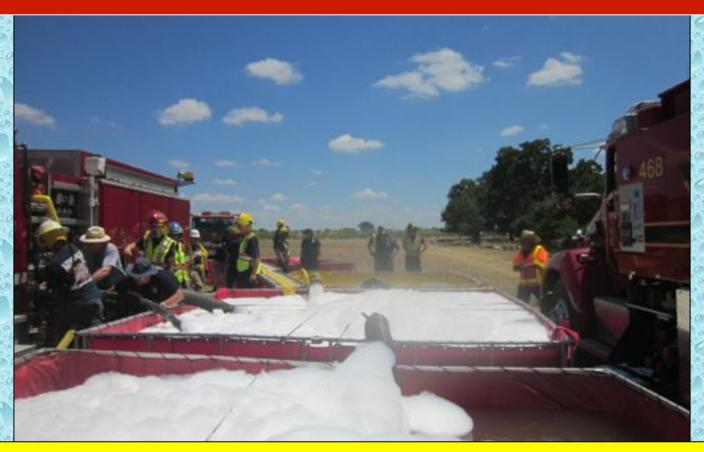
Around the 30-minute mark, four dump tanks were down, but only two were in operation as crews waited to acquire more jet siphon devices.
