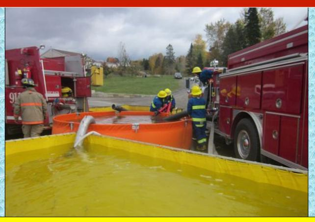
As the flow moved to 1,000 gpm, the dump site pumper began to struggle to run two jet siphons and flow 1,000 gpm. Adding the 2-1/2" suction line helped some, but the greater plan was to transfer the jet siphon operations to another unit.
