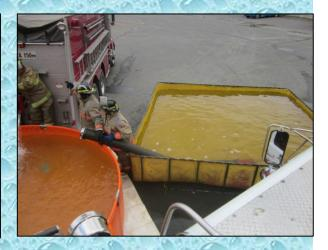
With three dump tanks in operation, the flow was moved to 700 gpm at the 30-minute mark and then to 1,000 gpm at the 45-minute mark. The three large dump tanks provided adequate "on-site" storage to support this size flow.
