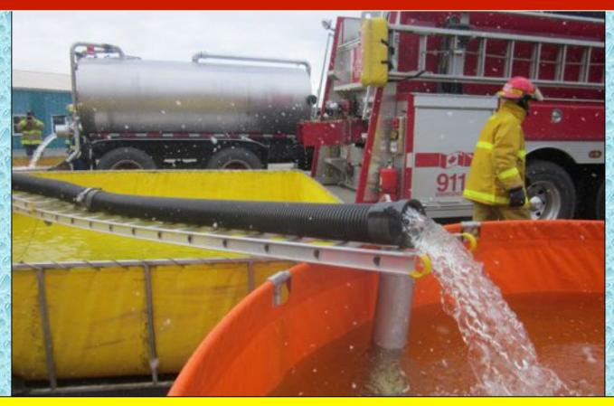
The three jet siphons easily supported the 1,000 gpm flow and the primary dump tank was kept full.
