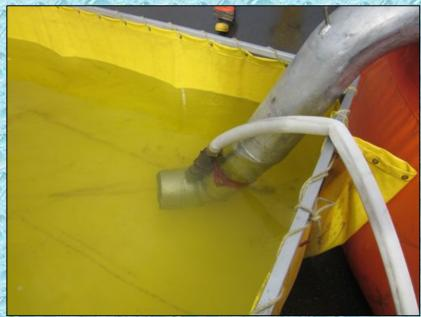
Water transfer operations were critical to the success of this drill. The 1,250 gpm was unable to flow 1,000 gpm and run three jet siphons (four dump tanks), so the decision was made to use portable fire pumps to run the jet siphons.
