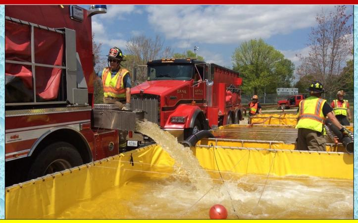
Around the 70-minute mark, work begins on setting up a fourth dump. Tankers are beginning to arrive back at the dump site at a more regular pace.
