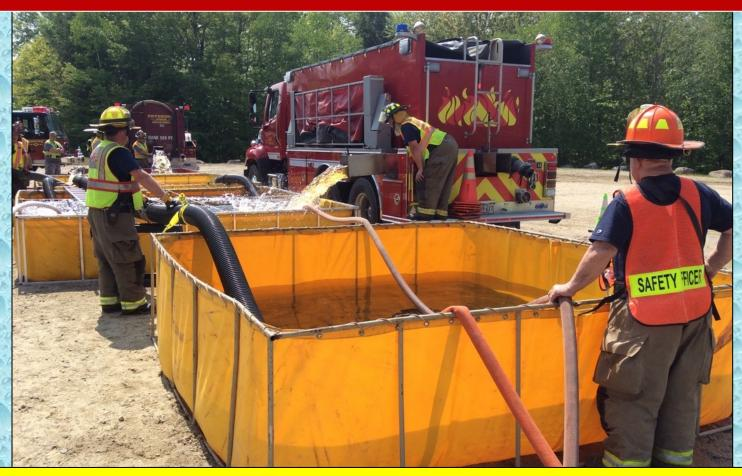
The four-dump tank operation was able to support a 1000 gpm flow starting at the 75-minute mark. That flow was sustained for the remainder of the drill.
