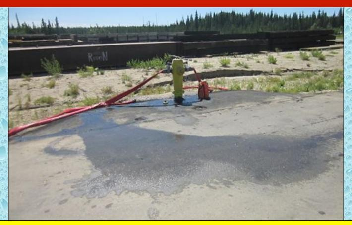
The second fill site used a fire hydrant without an engine. Tenders loaded directly from this hydrant using dual, 65mm lines.
