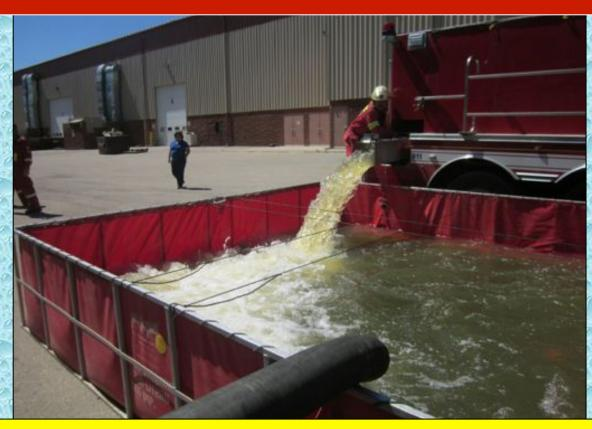
Tender 1701 arrived very shortly after the first engine. The tender's crew of two helped deploy the 3,500-gallon dump tank. Once Engine 1402 was ready to draft, Tender 1701 dumped its 3,500 gallons of water into the dump tank and left for the fill site. At the 5-minute mark, water flow was started at 300 gpm.
