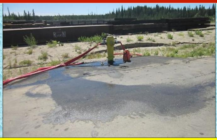
At this fire hydrant, the tender crews simply loaded their tenders directly off of the hydrant using two, 65mm lines. This site was not as fast as the second fill site, but the fill rate was respectable.
