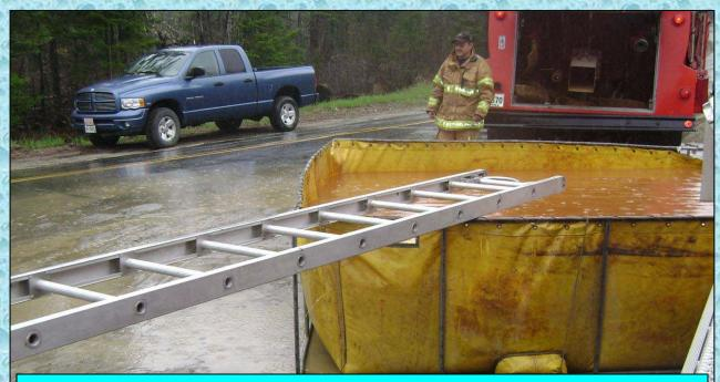
A roof ladder is used to bridge the gap between two of the three tanks. By spacing out the one tank, space is gained to allow more than one tanker to get into position to offload.
