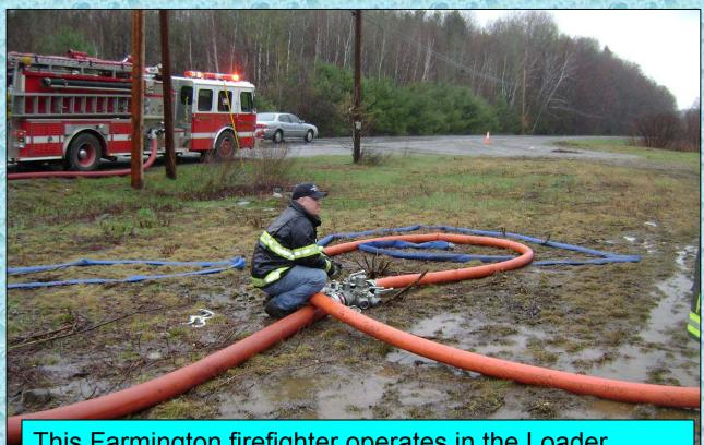
This Farmington firefighter operates in the Loader position and operates the LDH manifold that controls the flow of water to the tanker.
