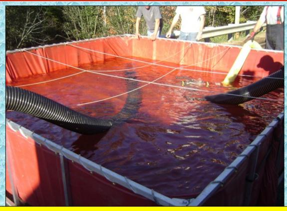
Had the portable pumps been connected directly to the supply pumper, cavitation of the supply pumper most likely would have occurred. But...by feeding the dump tank from the portable pumps, the supply pumper was able to draft and support a much higher flow rate.
