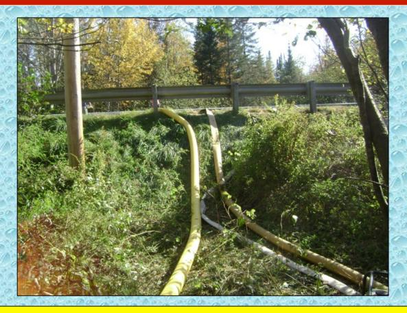
Each of the portable pumps discharged their water up a short incline through 100 feet of 5-inch LDH.
