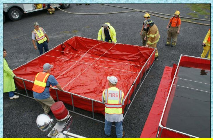
With more tankers arriving, another dump tank is set-up. Sylvania Engine 2's 3,000-gallon dump tank is shown above being set up.
