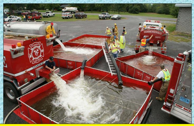
With the flow now at 1,000 gpm, crews were kept busy running a 4-dump tank operation.
