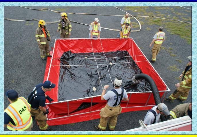
While the Adamsburg tanker is pumping its water to the attack engine, crews set up the tanker's 3,000-gallon dump tank.
