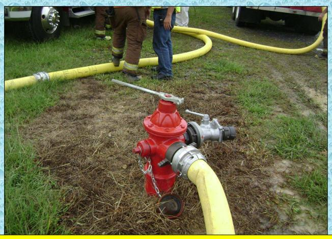
By putting a valve on one of the outlets, additional water can be obtained without having to shut down the hydrant.
