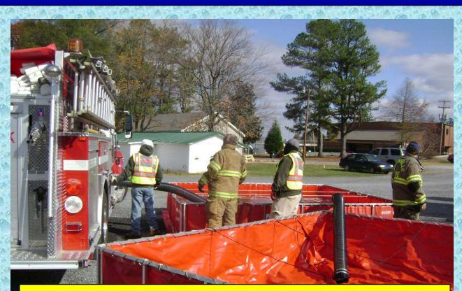
With water now flowing, Kilpatrick Engine 2 arrives and the first dump tank (3,000-gallon) is set-up.
