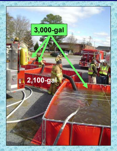
A 4<sup>th</sup> dump tank (3,000) is set-up and the dump site becomes fullyoperational.
