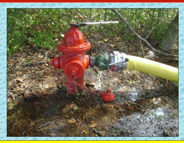
To increase the ability of the hydrant, a 5-inch line is used to fill a dump tank from which Sylvania Engine 2 (1,250 gpm) drafts and fills tankers at 1,000 gpm.
