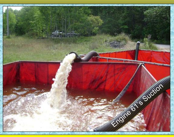
With the second dump tank operational, the flow is increased to 500 gpm at the 40:00 minute mark. However, crews continued to struggle to support the flow as it seemed that water was being used as fast as it was being dumped.
