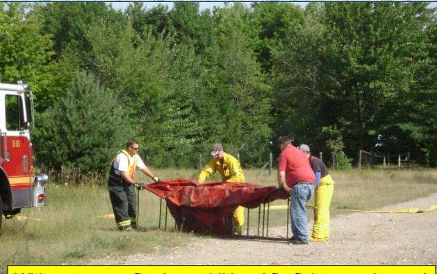
With water now flowing, additional firefighters arrive and the first dump tank (2,100-gallon) is set-up.
