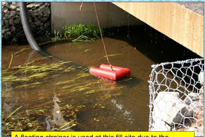
A floating strainer is used at this fill site due to the amount of aquatic vegetation.
